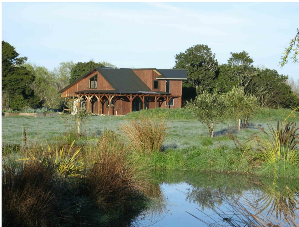
Figure 7 House on lot 1 under construction
